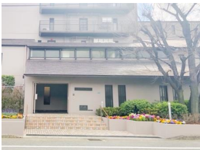
In front of the dormitory building
